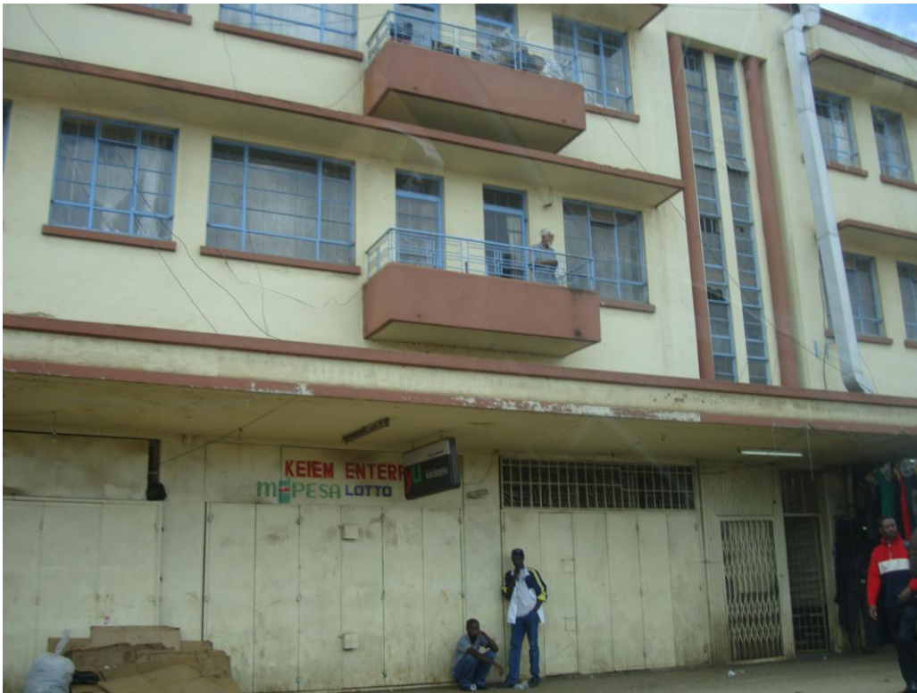
Building at corner of Ngara Road at the far end. Note: the Muhindi gentleman at first floor balcony and the seedy atmosphere below.
